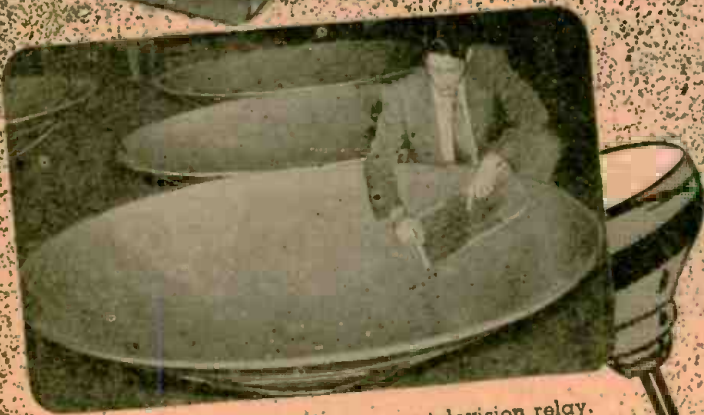
Fig. 3 - "Big Dishes" for microwave television relay. Devised by General Electric Co. engineers for reflecting television signals between relay stations.
