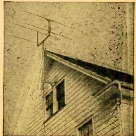
Two-deck television antenna with reflector, commonly used in remote receiving locations.
